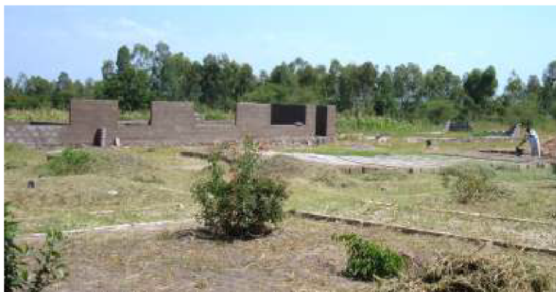
New Secondary School laboratories and library walls going up
