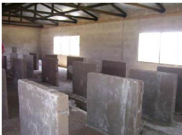
Inside lab building, getting ready for lab tables, sinks, plumbing, etc.
